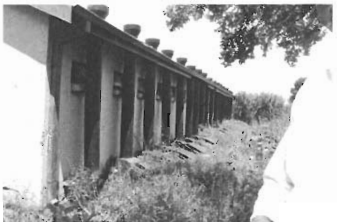
ENVIRO LOO SYSTEM USED IN OLD ABLUTION FACILITY
