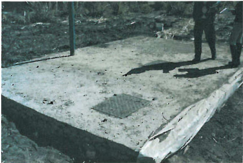
NEW SEPTIC TANK
