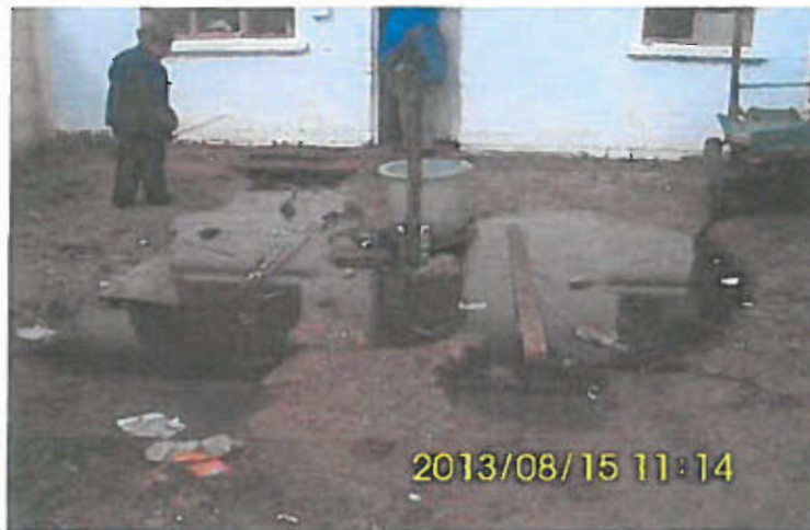
Photograph 3 depicts the circuitous route which has to be followed in order to access the houses.
